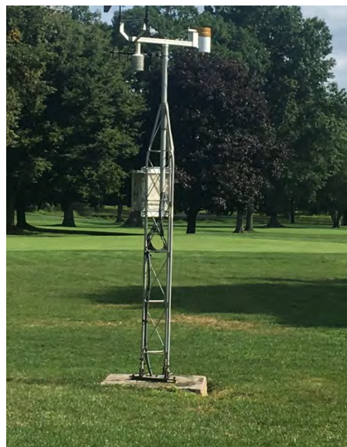
Figure 6. On-site weather stations provide the data for more precise irrigation control.
