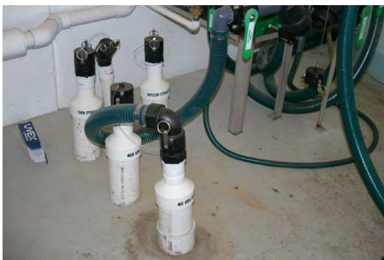
Figure 22. Equipment mix and load area with recovery lines.
